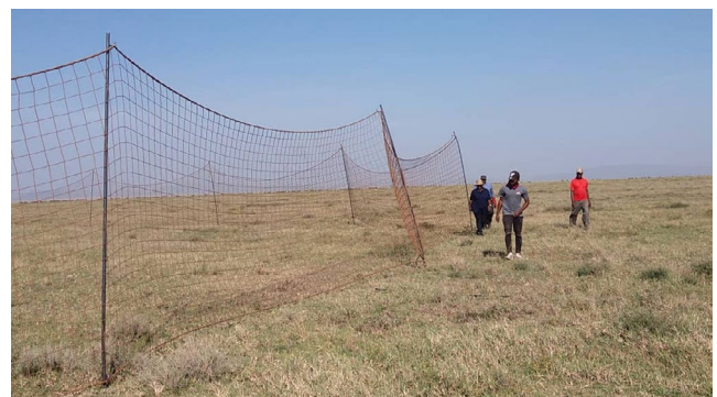
FIGURE 2 Picture showing netting structure with pipes inserted into ground pinned metal bars and hanging nets [Colour figure can be viewed at wileyonlinelibrary.com ]
